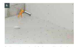
Apply a continuous bead of solvent weld to the edge of the shower base, as shown. Lay the first panel onto base and against the wall applying pressure to ensure the panel is fitted firmly against the base. Secure the panel in place using drywall screws at approx. I 50mm centres into the stud-work, then wipe clean surplus solvent weld.
