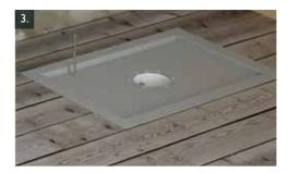
Mark centre lines of exposed joists onto flooring. Insert metal tray into cut-out and transfer drawn lines onto tray. Drill and countersink two holes per joist through metal tray to suit csk-head wood screws (not supplied). Screw metal tray into position.
