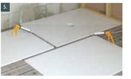
Using KUDOS Solvent Weld, apply a continuous bead to the edge of the shower base, as shown. Lay the first aqua4ma panel up to the edge of the base applying pressure to ensure the panel is fitted firmly against the base edge. Secure the panel in place using drywall screws at 150mm centres, then wipe clean surplus solvent weld. Joints should be staggered, as shown to help strengthen the overall assembly.
