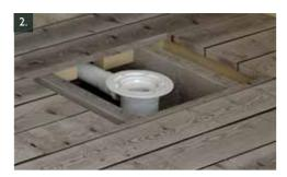
Using circular saw, saw depth to suit floor thickness and remove the area of floorboards. Connect waste body using 50mm/2" solvent weld waste pipe (not supplied), ensuring waste body is positioned to centre of the cut-out. Screw fix 4" x 2" (100 x 50mm) timbers (not supplied) to underside of flooring to strengthen the edges of the cut-out.
