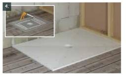
Apply beads of KUDOS Grabber Adhesive to base of metal tray and the 4 outer flanges as shown. Carefully position shower base into position and stand on it to ensure it is fully bedded down onto tray and floor. Secure in place by using drywall screws (not supplied) around the perimeter at 150mm centres ensuring these avoid the metal tray underneath.
