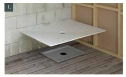
Place shower base in required position against wall/s and mark position of centre waste hole onto flooring. Remove base and position metal tray ensuring waste hole is centred over marked position. Mark corners of tray onto flooring. Measure and draw lines inside of marked corners, this is the area of flooring to be removed.
